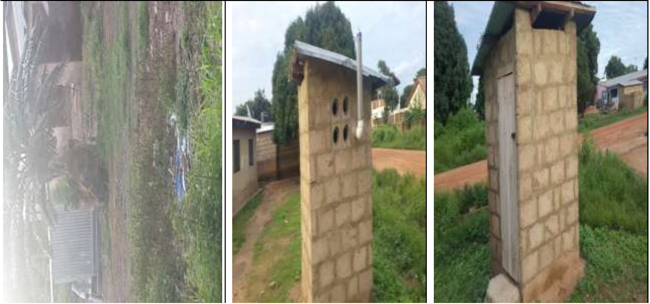
Figure 5. Detached KVIP toilet facilities; Household toilet facility detached from a compound house and L-shape building. All zinc built toilet facility is behind the L-shape house while the cement block and zinc roof toilet facility is found outside a compound house.
